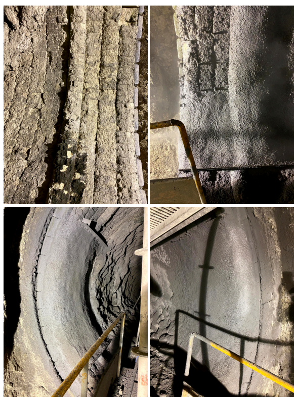
Turkey: Old brickwork outlet zone, before and after installation with REFKO Recovery MG 78.
