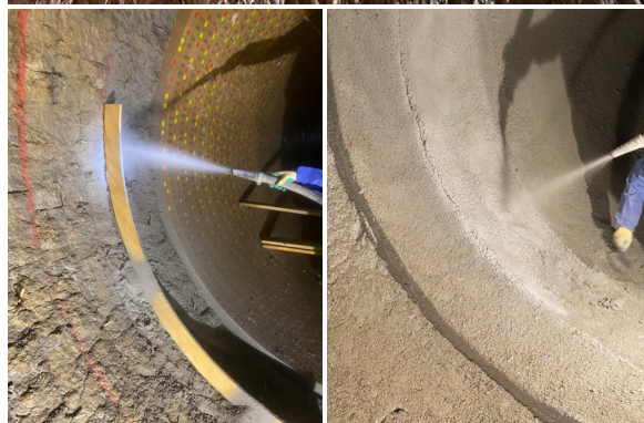
North Rhine-Westphalia: (top) old brickwork, almost dust-free gunning with field classification. (Bottom) final result after installation.
